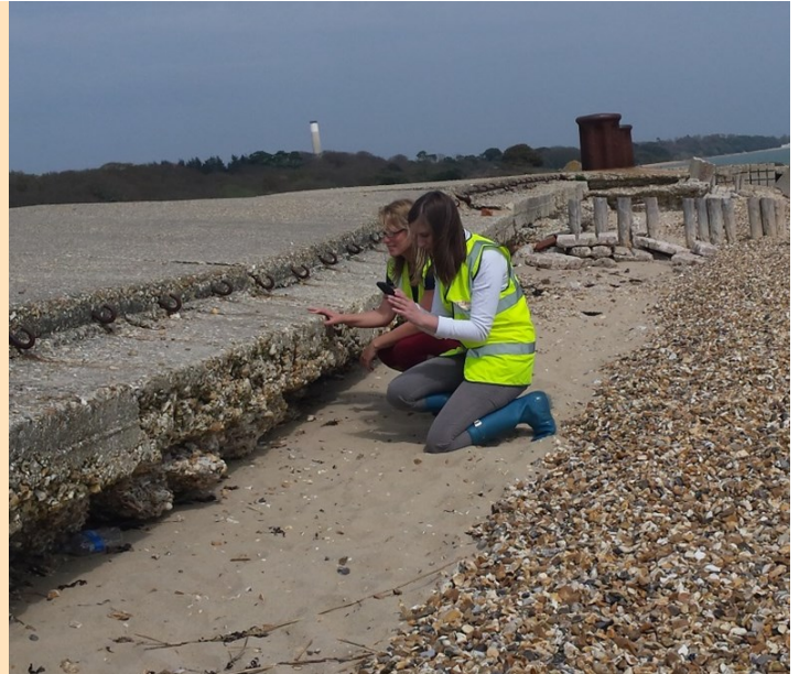
Work on the seafront with the D-Day remains at Lepe
