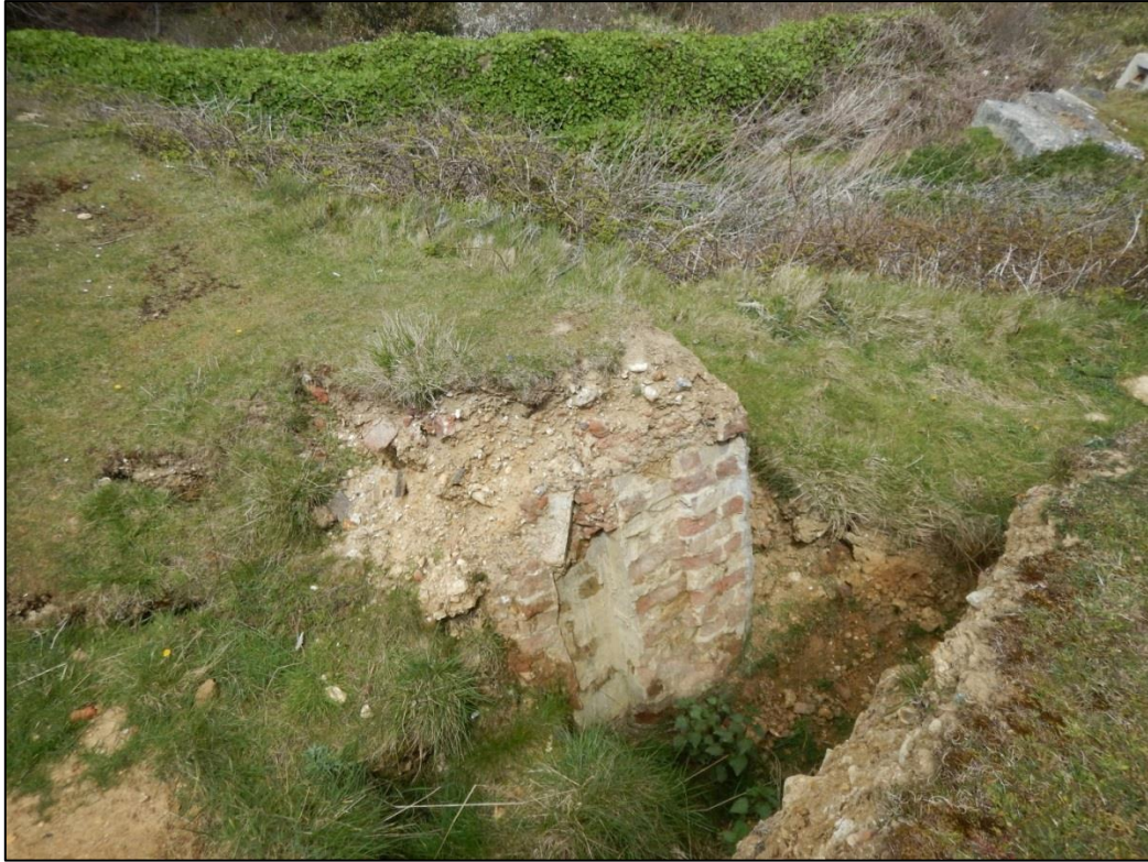
Figure 15: Looking north over some masonry remains of A Group which has slumped down, in the top right of the picture remains of Gun 2 of A Group are visible.
