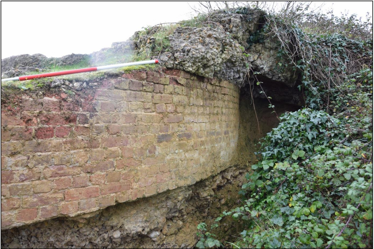
Figure 19: Masonry structures eroding out of cliff, camera facing south-east.
