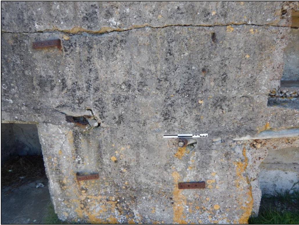
Figure 39: Looking west, pipework under C Group.
