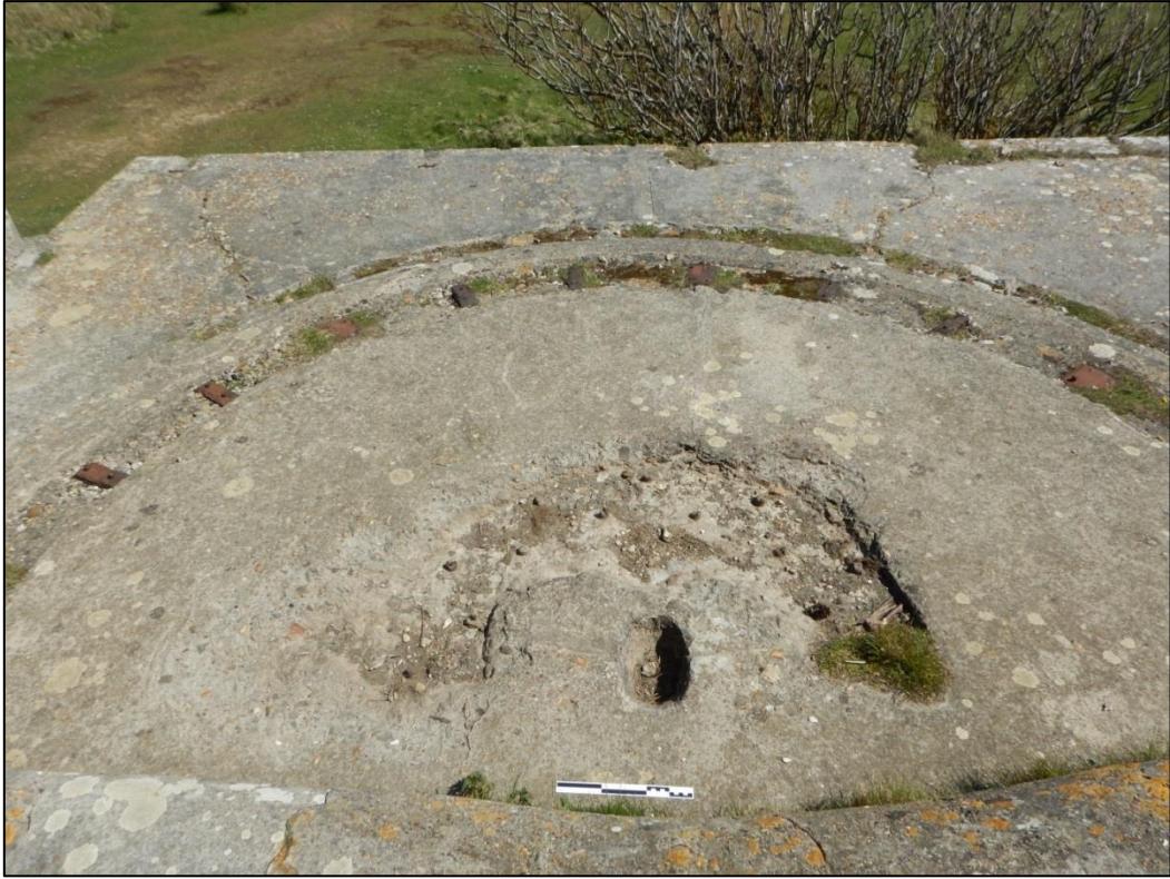
Figure 43: Looking east/north-east over the base which would have been gun 2 of C Group.
