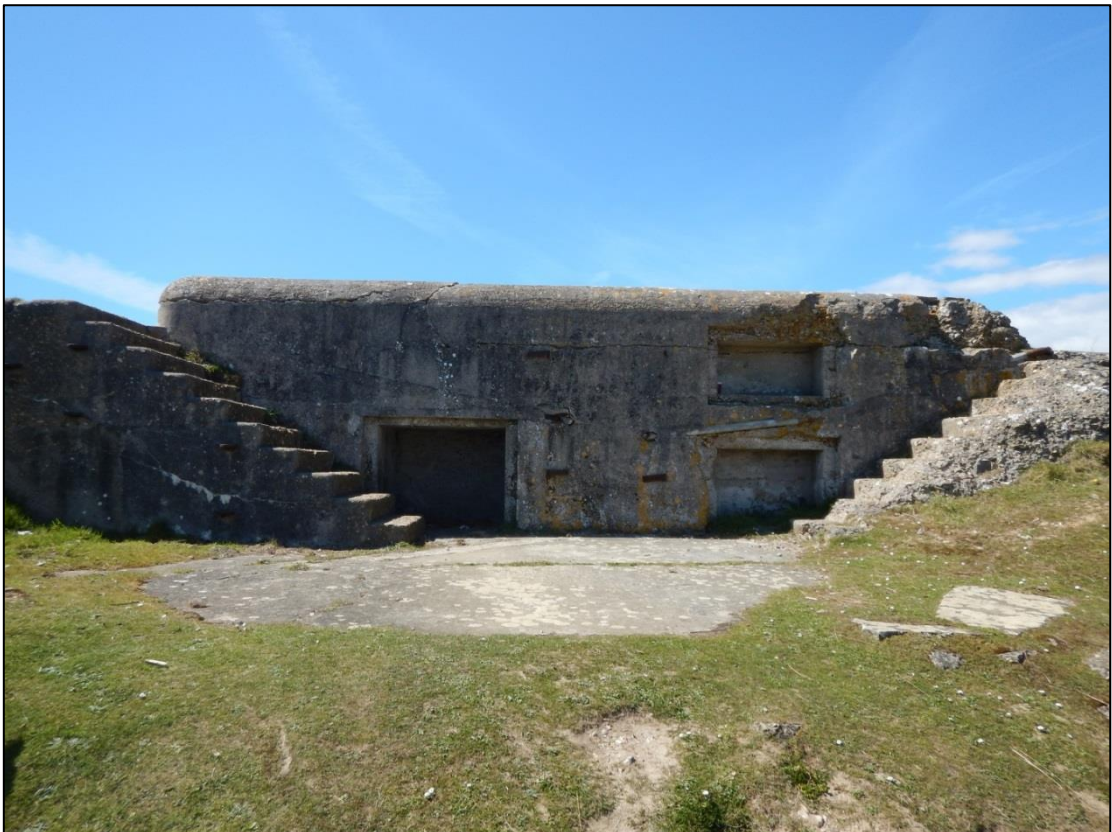
Figure 34: Close up of C group, looking west/south-west.
