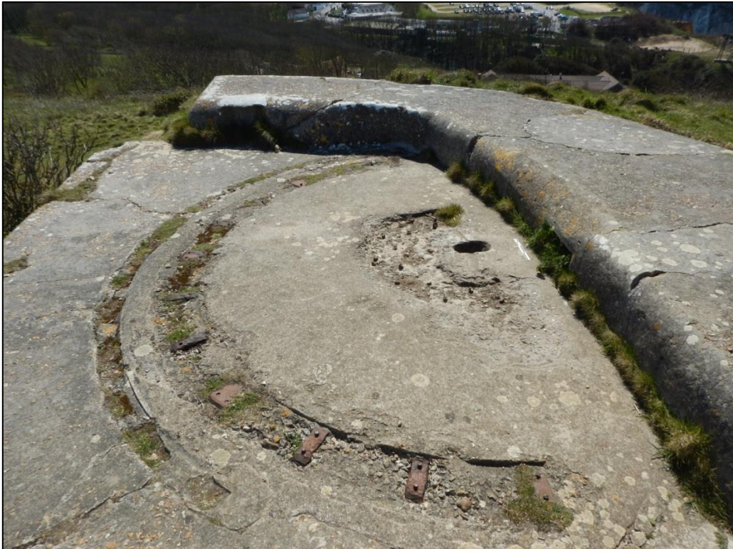
Figure 44: Looking south over Gun 2 of C Group.
